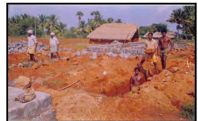
Construction of New House in
